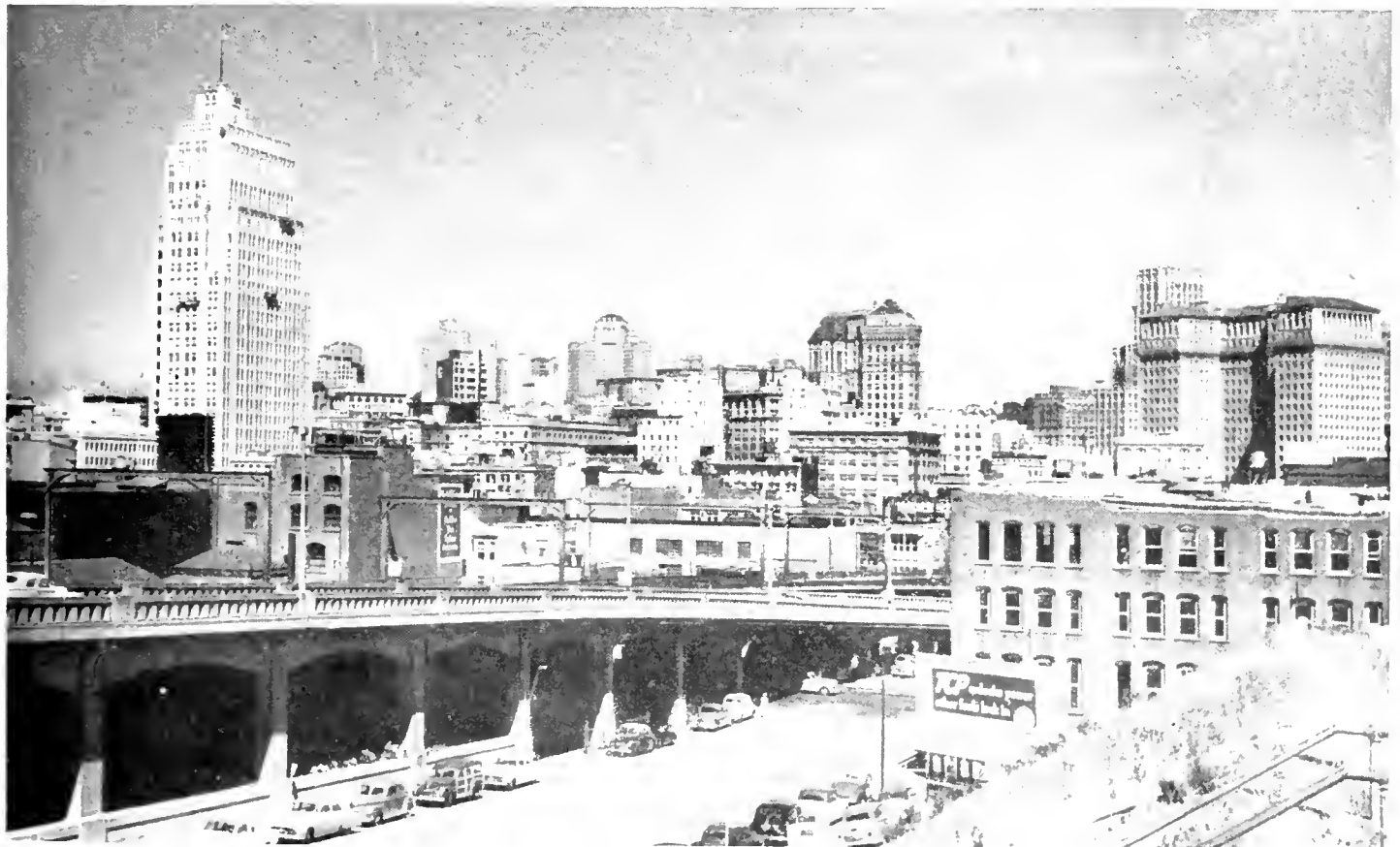
First Street off-ramp for dispersal of Bay Bridge traffic into commercial and financial districts
